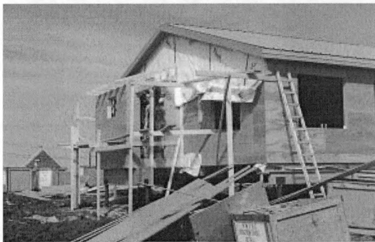
Exterior of a housing unit nearing completion.
