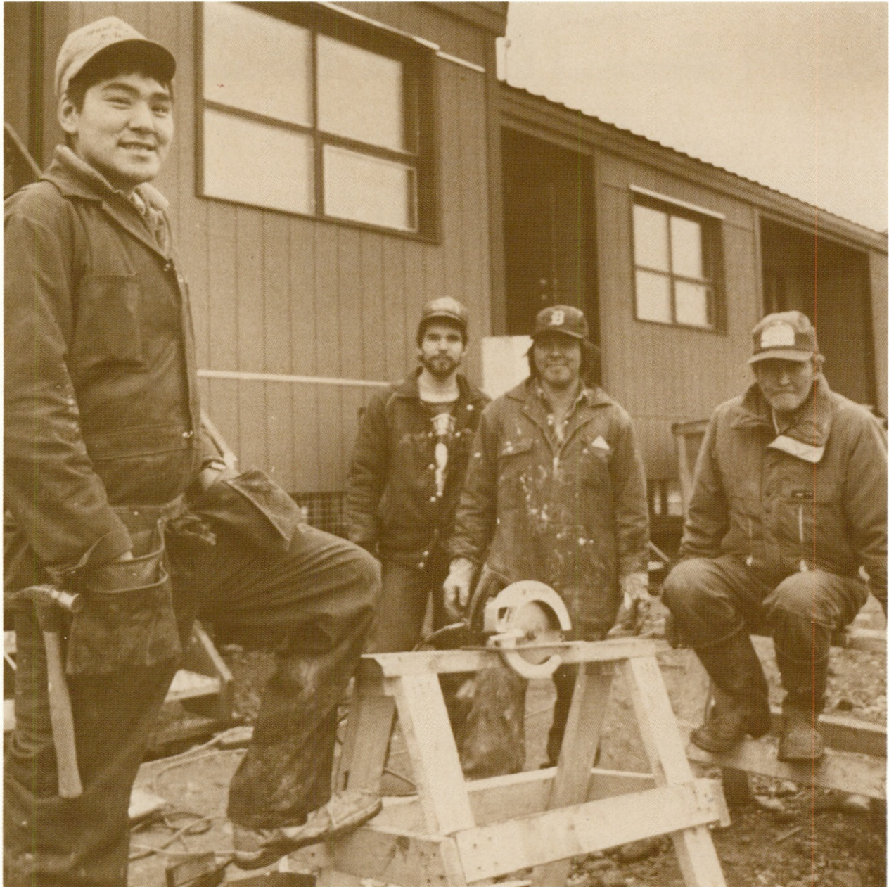
Public Housing Construction, Aklavik. Tom Elanik, Shawn Reed, Walter Malagana, Walter Bennett. (Macintosh.) ᑭᑭᑕᑕᑦ ᑕᑦᑕᑕᑦ ᑕᑦᑕᑕᑦ ᑕᑦᑕᑕᑦ, ᑕᑦ ᑕᑕᑕᑦ, ᑕᑦ ᑕᑕᑦ, ᑕᑕᑕ ᑕᑕᑕ, ᑕᑕᑕ ᑕᑕᑕ. (ᑕᑕᑕ.)
