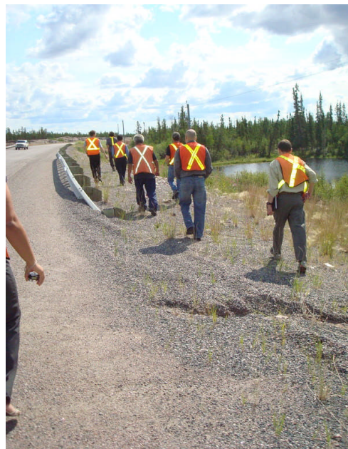
PIEVC Workshop participants on a site tour of Highway 3 (photo DOT)
