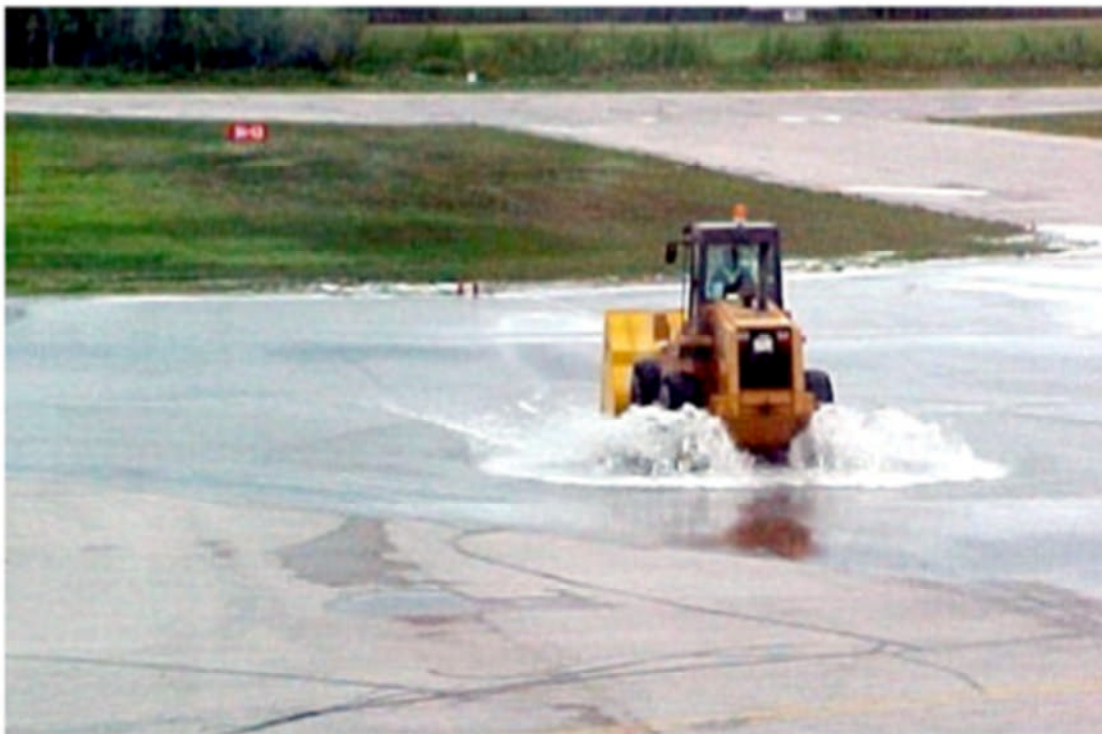
Figure 5-2 Inundation of the apron surface at Hay River Airport
