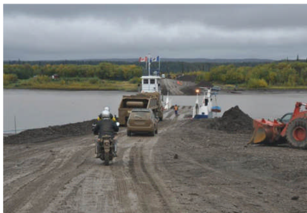
Loading ramps and vehicle staging areas are constructed from gravel and are an adaptable system. Future adaptation might require more permanent drainage.
