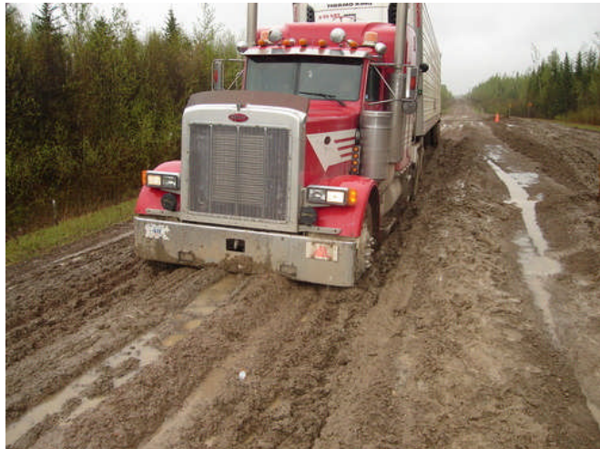
Wet conditions on the Liard highway have caused spring closures in recent years (photo DOT)
