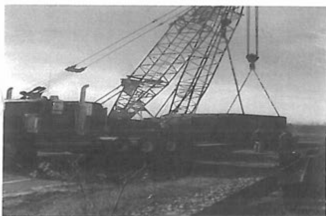
M200 North getting removed from truck to load onto rail car at CN rail yard
