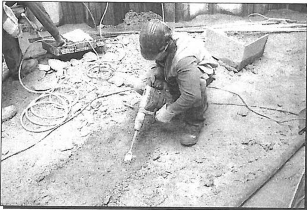
Photo 3 Pier 1 (preparing footing for drilling)
