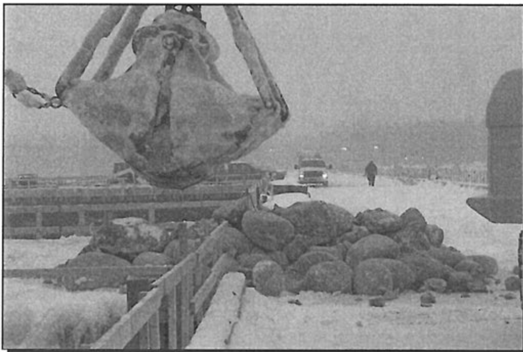
Photo 4 Buckets attached to crane for placing the scour rock into the cofferdam
