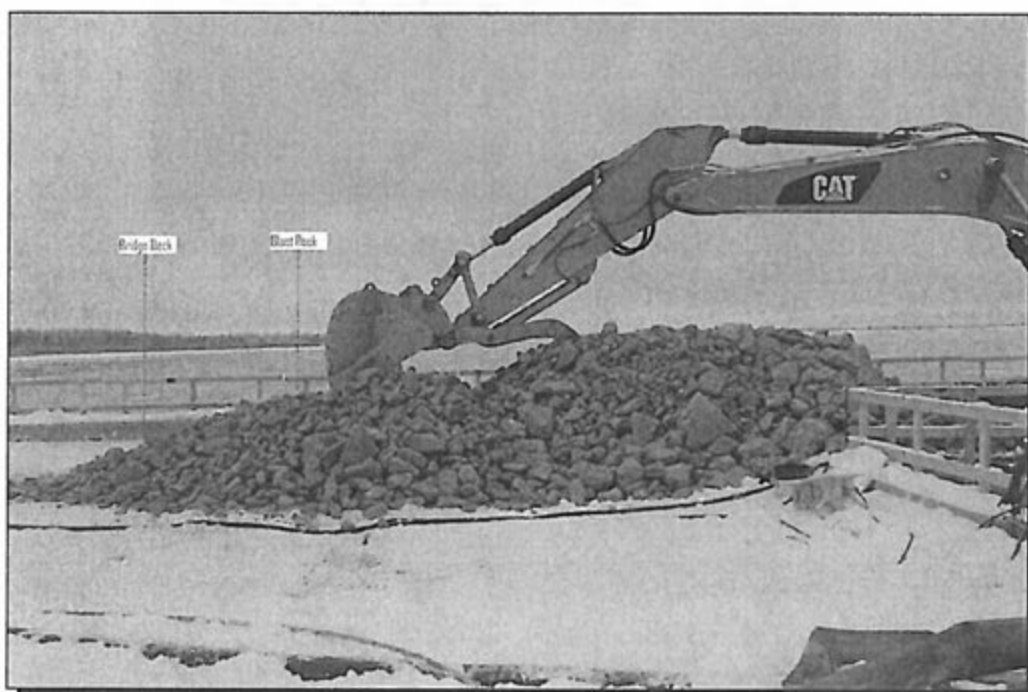
Photo 4 Blast rock delivered to Pier 2 South, on the temporary bridge deck.
