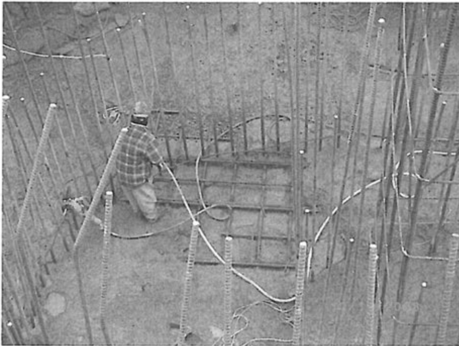
Photo 2: Concrete removal in progress, October 17, 2008. Note that the depression extends outside the dowels for the lower buttress. This could be either the northwest or southeast corner.
