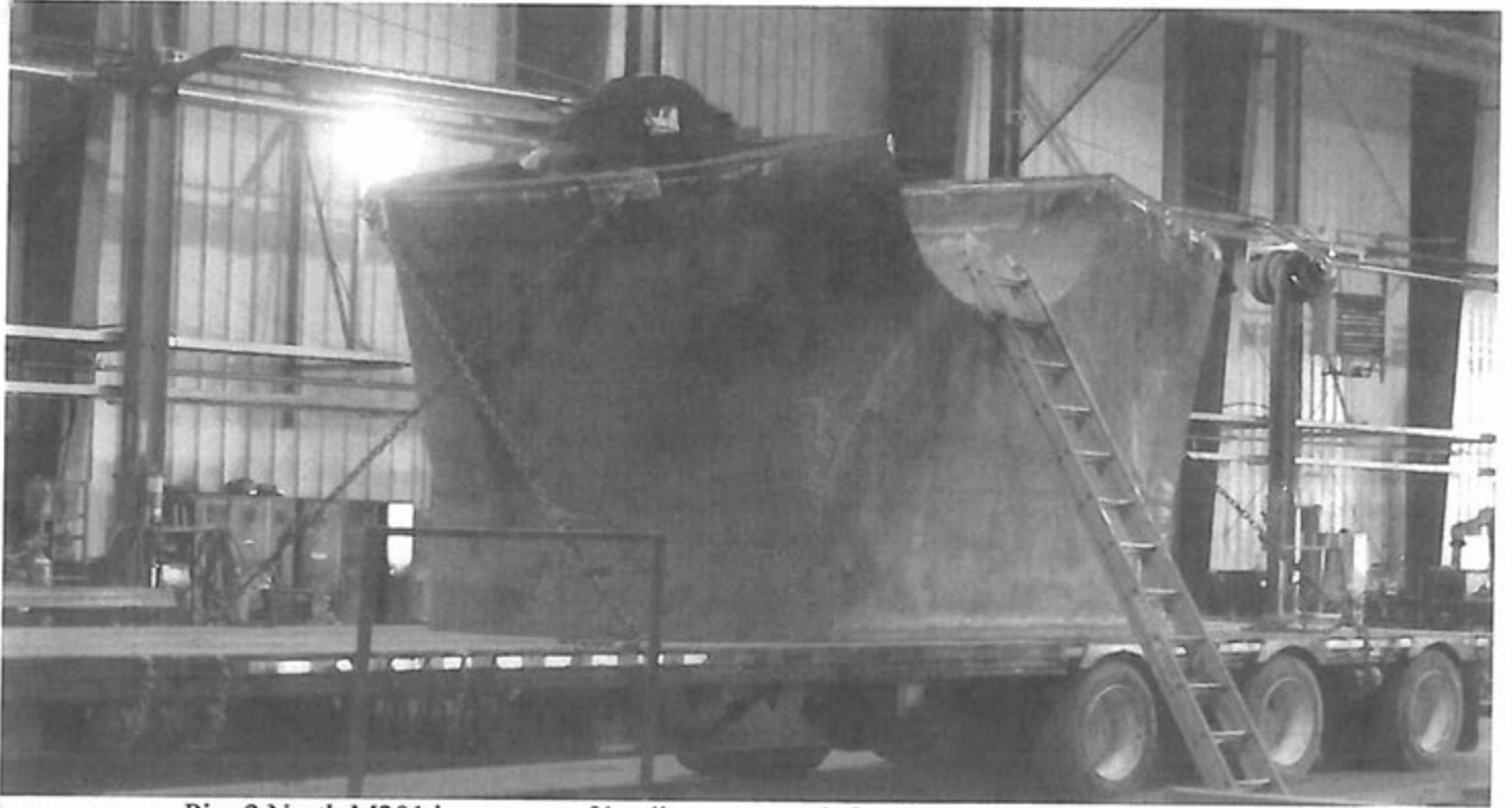
Pier 2 North M201 in process of loading onto truck for transport to site at Yellowknife
