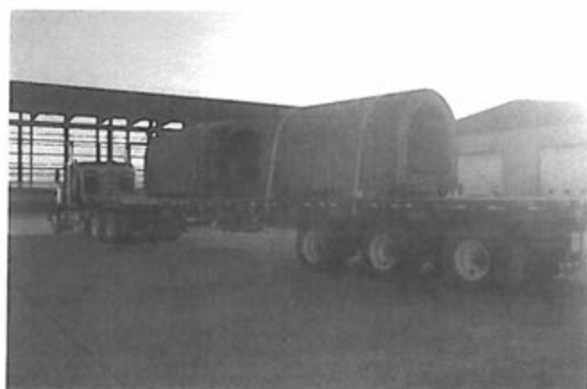
Pier 2 North M202 loaded onto truck for transport to site at Yellowknife
