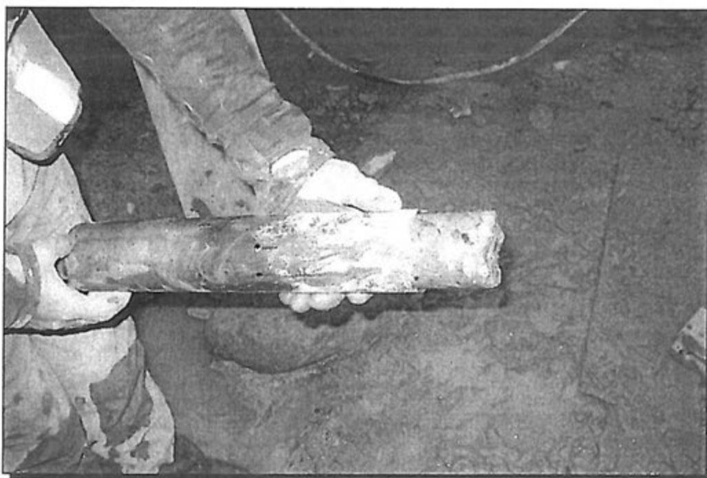
Photo 6 Pushing out concrete core
