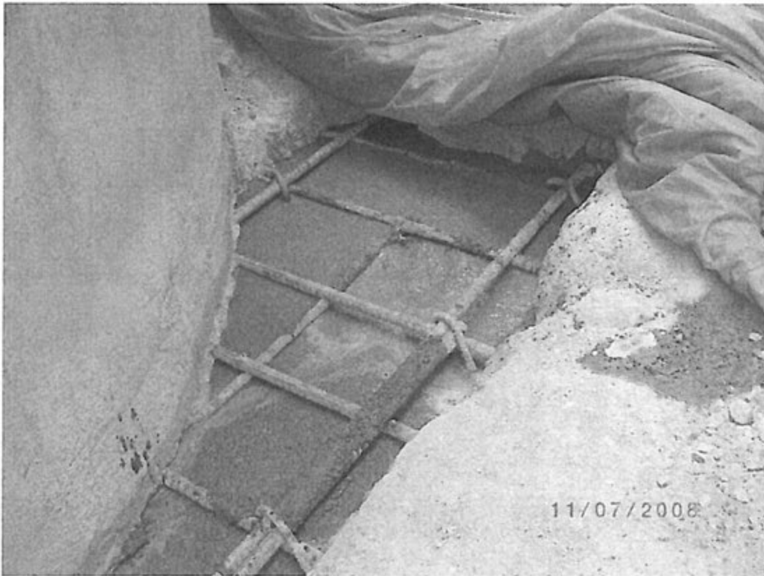
Photo 1: Depression partially filled with fresh concrete, November 7, 2008. This could be either the southeast or northwest corner of the Lower Buttress.
