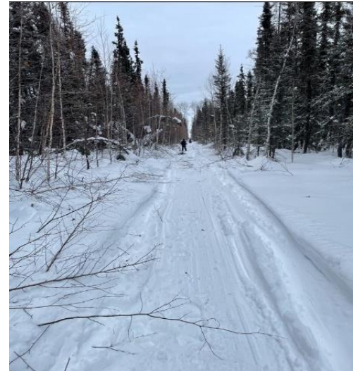
Access trails continuation construction - Nahanni Butte.
