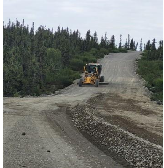
Grading operations as part of Summer 2021 continuation construction on the Wekweètì Access Road.
