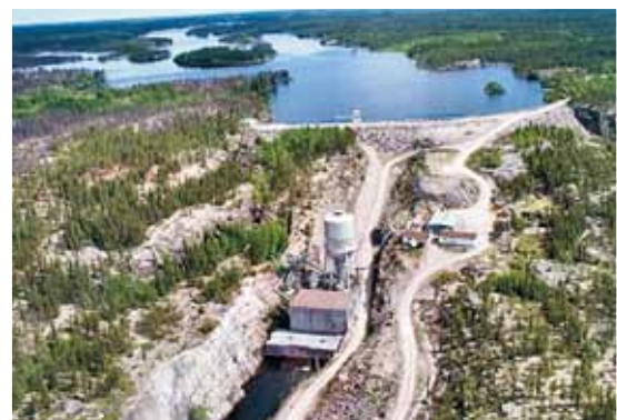
Taltson Hydro Dam
