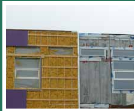
Prototype section of the building has been spray foamed and strapped, exterior cladding is being applied.
