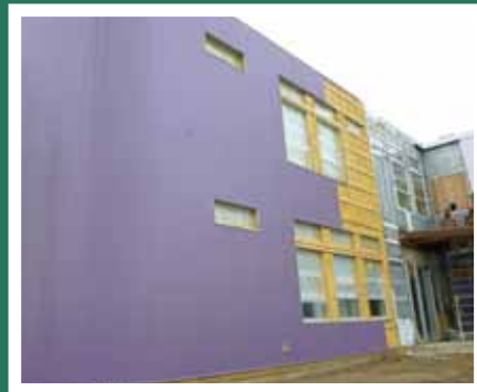
Particular attention was paid to how the new envelope was constructed at corners and fenestrations and how connections were made at parapets and footings.
