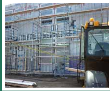
Contractors have removed the existing “skin” of the building and are beginning to apply the spray foam to the prototype section of the school.
